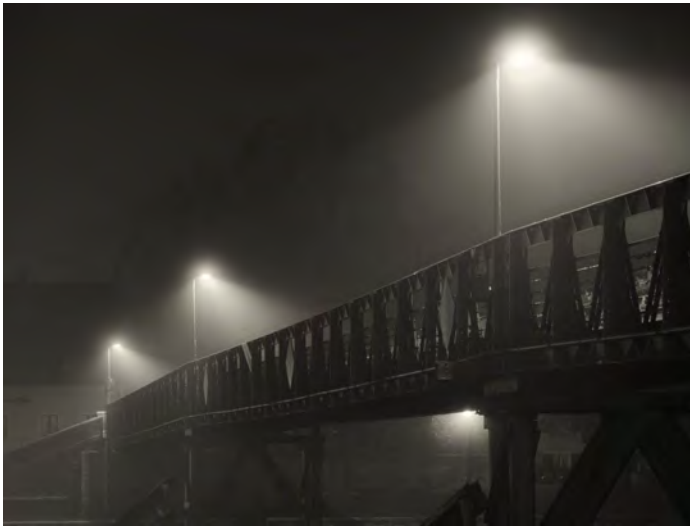
Vietnamese LED Street Light Lighting Project ▲
