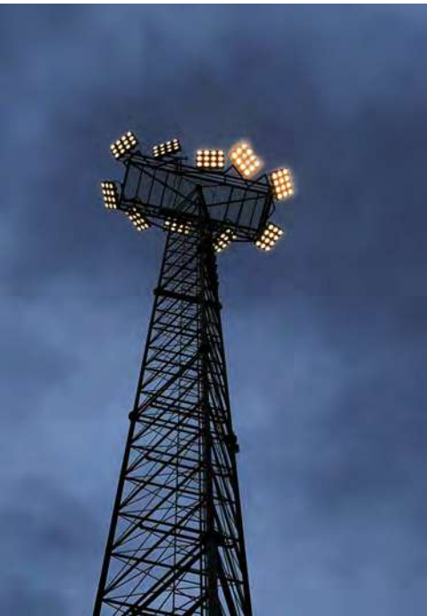
Belgian Dock LED Lighting Project ▼
