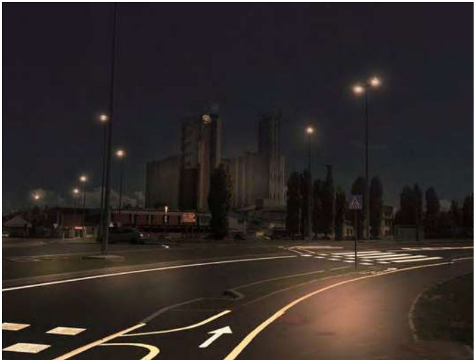
Philippine LED Street Light Lighting Project ▲
