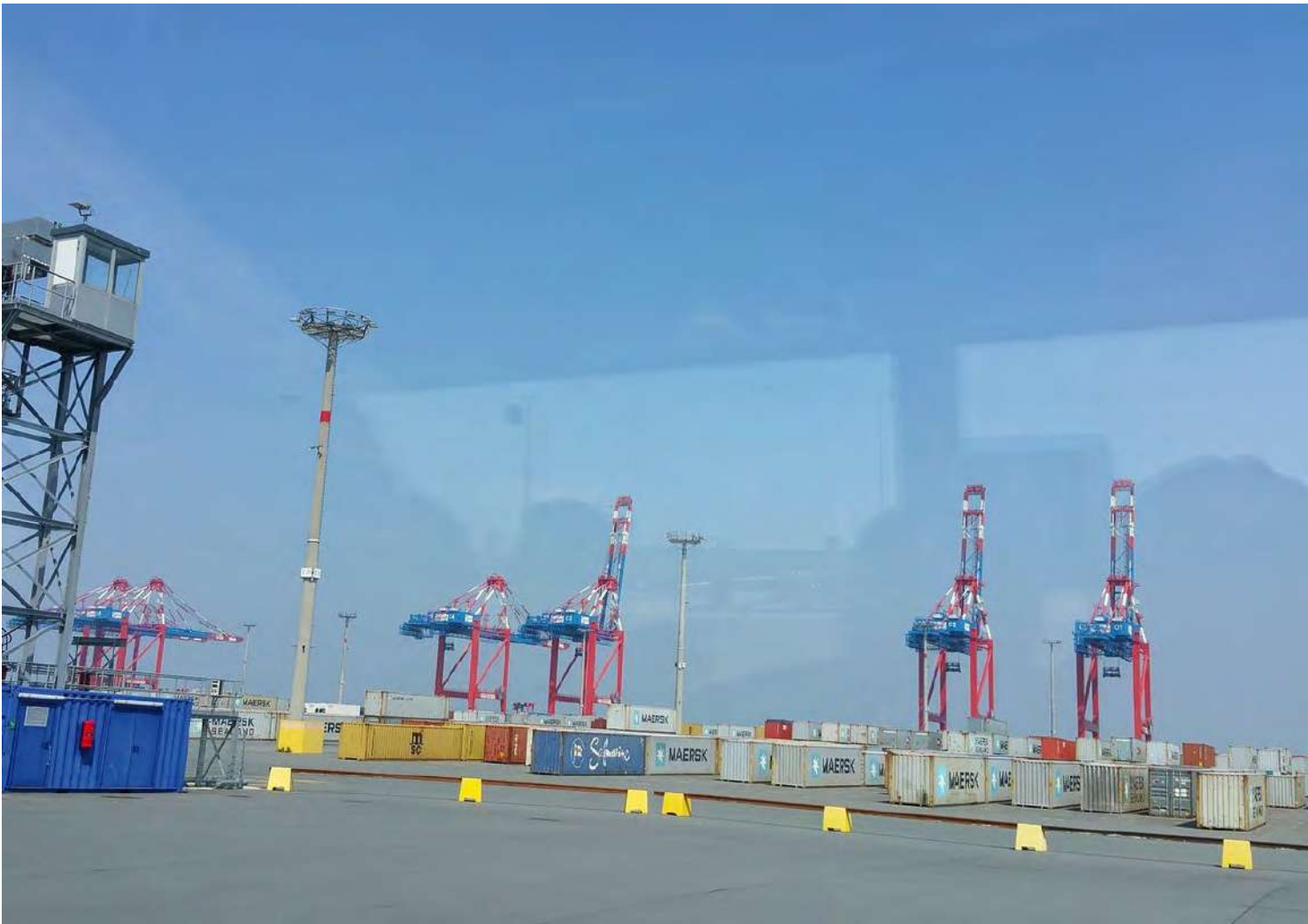
German Port LED Lighting Project ▲
