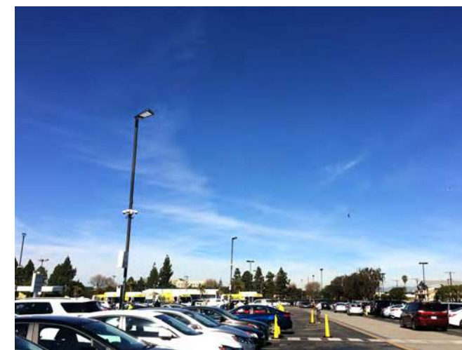
Spanish LED Parking Lot Lighting Project ▲
